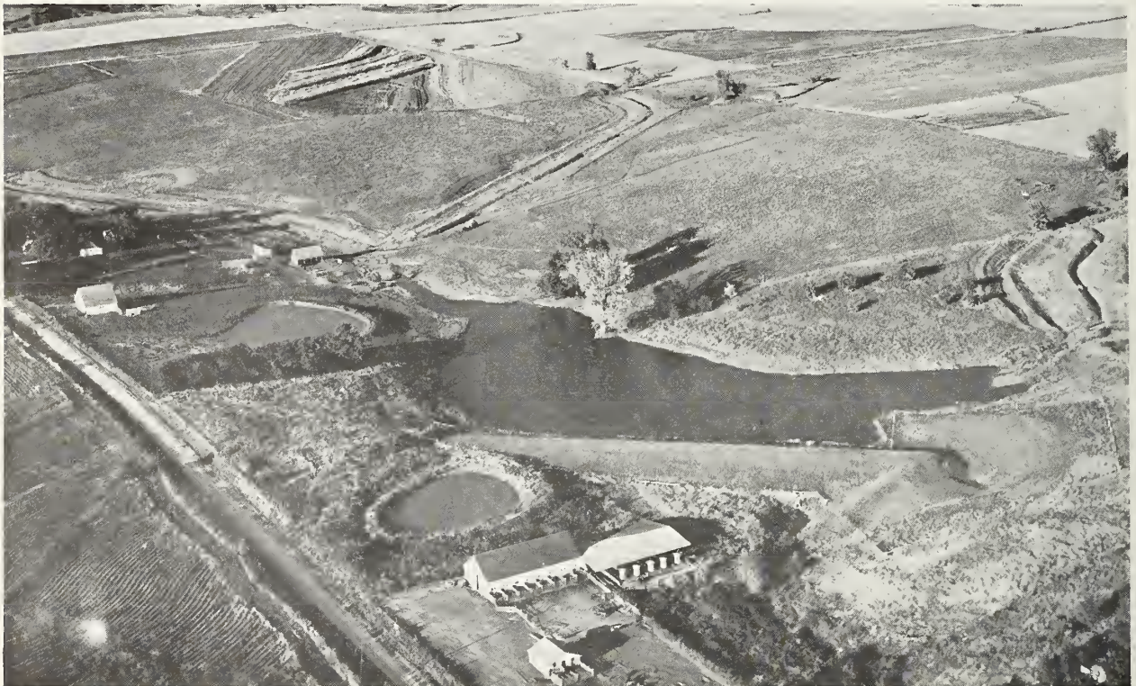
After project: Both land treatment and structural measures make an integrated watershed management program.
